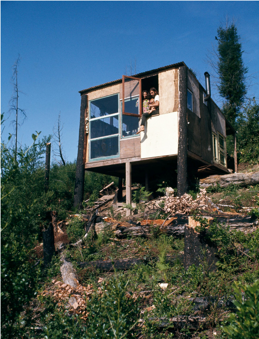
Figure 1. Joann, David, and their infant, Covelo Vishnu, in 1969 at The Chapel, their Wheeler's Ranch home built from salvaged lumber and windows, with trunks of redwoods that had been burned in an earlier wildfire serving as pilotis. Bob Fitch photography archive, © Stanford University Libraries
