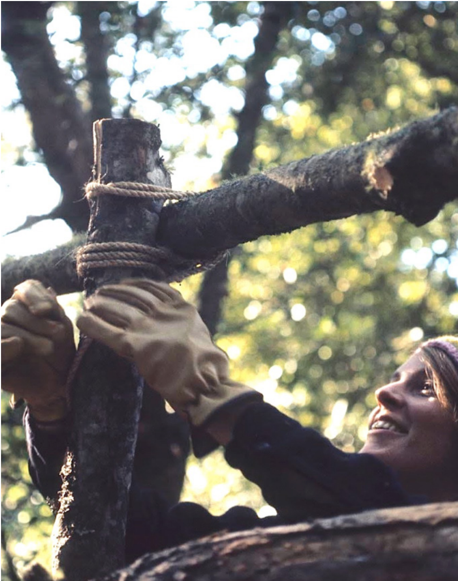
Figure 8. A Berkeley architecture student lashing together the frame for an individual sleeping cabin on the forested site of Arch 102ABC, the “Outlaw Builder Studio,” staged in Marin County during the 1971-72 academic year. Photo: Jim Campe, Jim Campe document collection, Environmental Design Archives, University of California, Berkeley.
